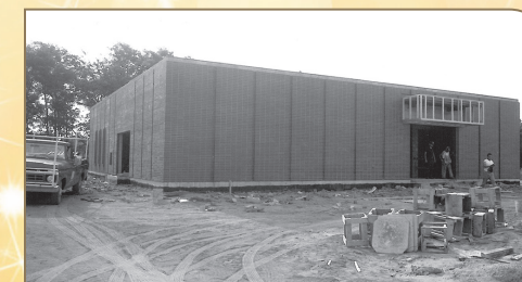
Burns Harbor Office construction, June 1977
